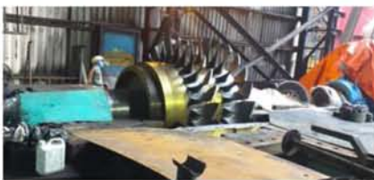
Rotor assembly checks in casing
