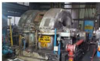
Turbine boxing up
